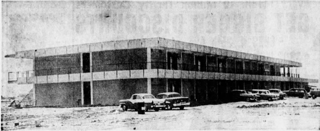
Bourgade High School, 31st Avenue And Hazelwood
